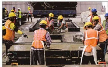
Started in September 2023, Kim is the largest track slab manufacturing facility.
